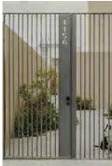
MT-1 STEEL FRAMES GATES NOM 50% OPEN (PEDESTRIAN & DRIVEWAY GATE)
